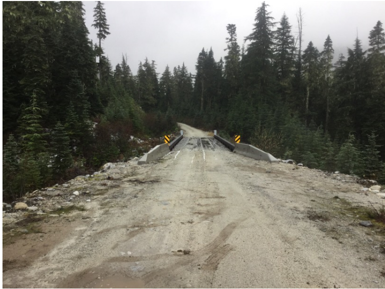
Approach from Right Bank when facing downstream
