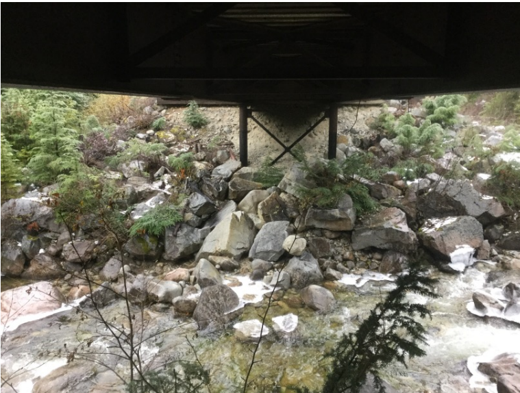
Right Bank Abutment when facing downstream
