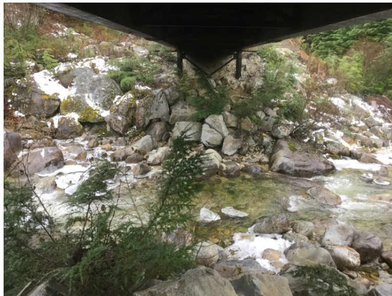
Left Bank Abutment when facing downstream
